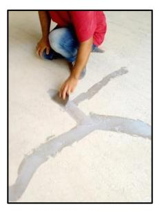
Surrounding areas should be covered and protected from material spills and equipment contact. Rope off work area. Cracks should be filled with a patching compound such as Crack Filler. However, it should be noted that some cracks might
