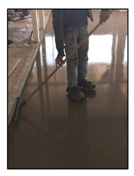
Cracks or joints in the existing substrate will reflect through the *GRANITOP-S* Stamp overlay. As in all flooring applications, the surface must be sealed for stain protection once the surface has cured for a minimum of 24 hours . If the *GRANITOP-S* Stamp topping is to be chemically stained, it must be allowed to cure for a minimum of seven days.
