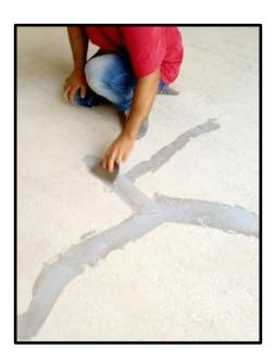
Surrounding areas should be covered and protected from material spills and equipment contact. Rope off work area. Cracks should be filled with a patching compound such as Crack Filler. However, it should be noted that some cracks might be moving cracks and could therefore cause reflective cracking in the *GRANITOP-M* thin layer. Any surface
