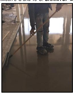
can be applied in thicknesses ranging from featheredge to 10 mm. A minimum application thickness of 2 mm is recommended. Use a gauge rake spreader to place the material, then follow lightly with a trowel depending on the desired final look. Do not over trowel. All mixed material must be used immediately. Timing is critical for proper spreading of the surface. Drying & curing time is 4-6
